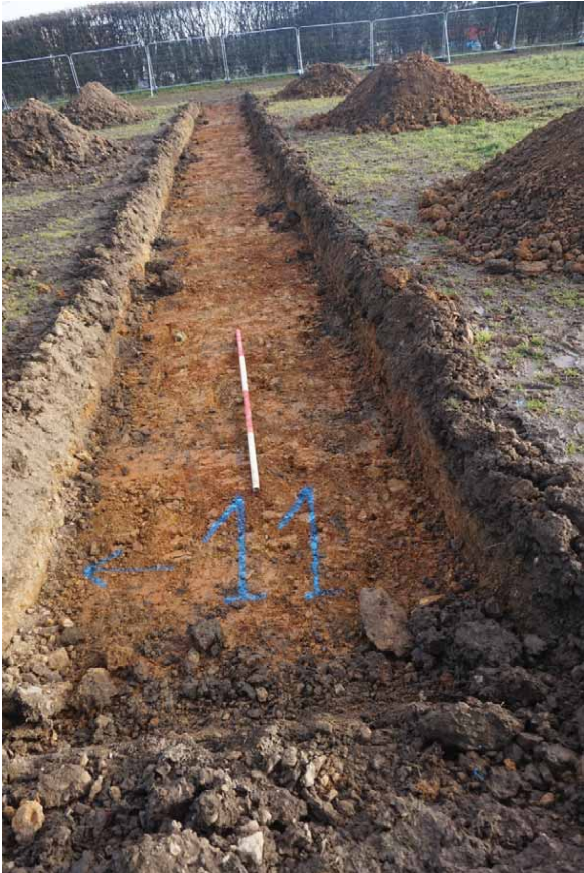
Plate 16: Showing Evaluation Trench 11. Looking east, two-metre scale.
