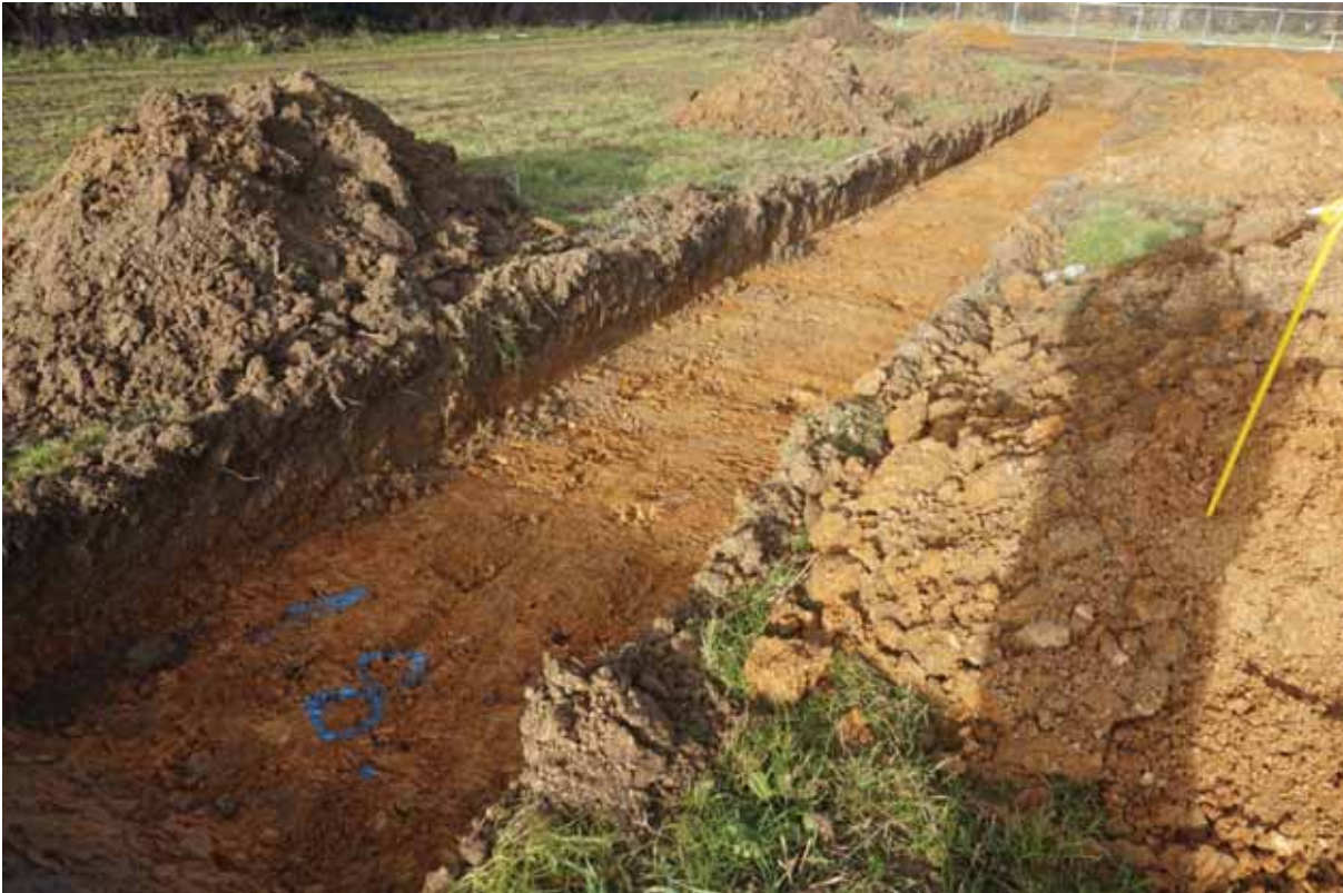
Plate 12: Showing Evaluation Trench 8. Looking north west, two-metre scale.
