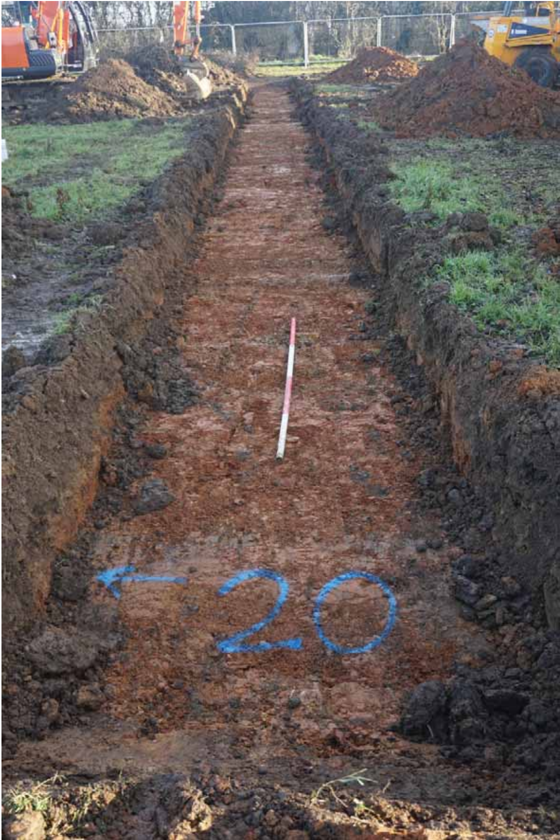
Plate 25: Showing Evaluation Trench 20. Looking east, two-metre scale.
