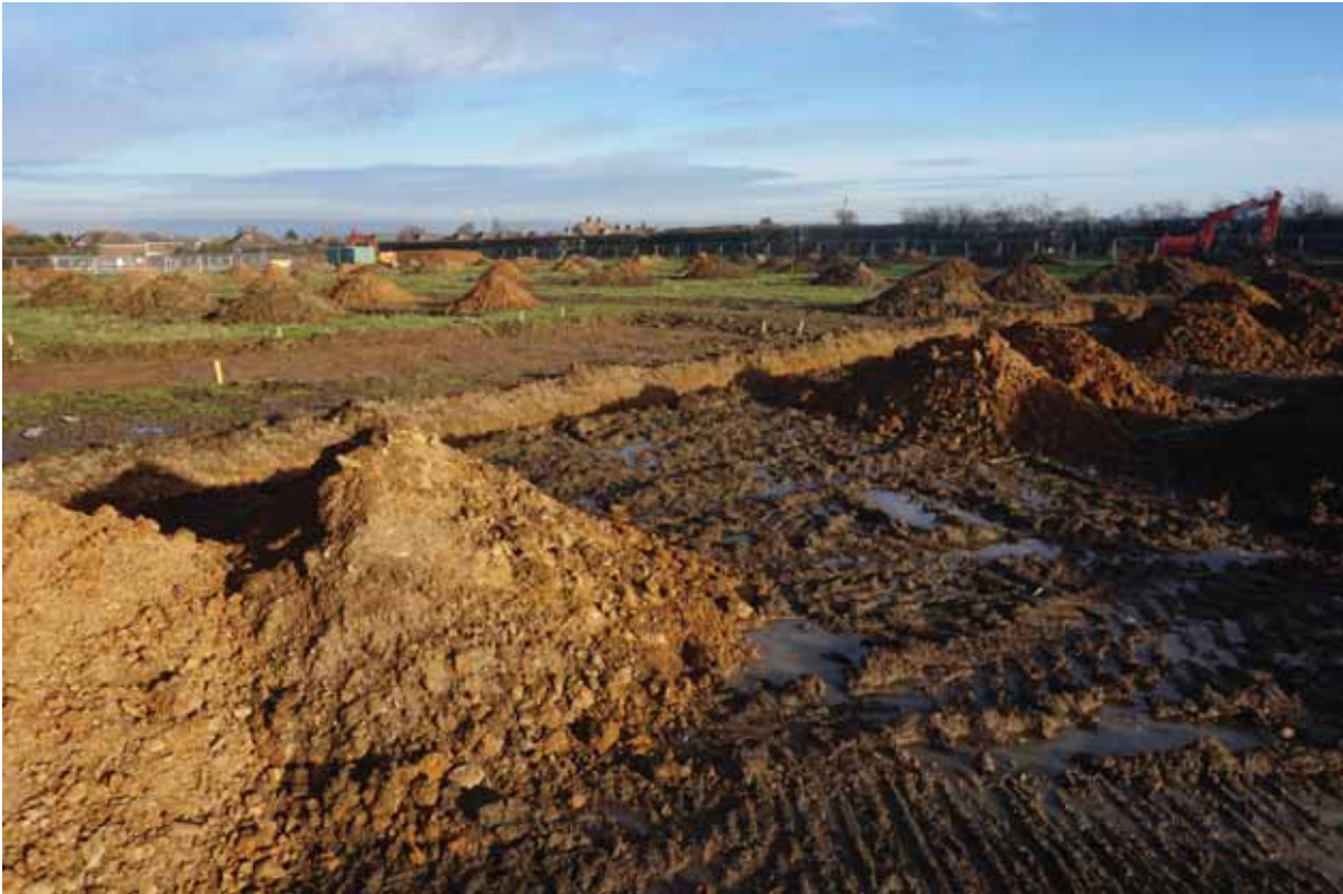
Plate 1: The site, looking north east from SW site corner.
